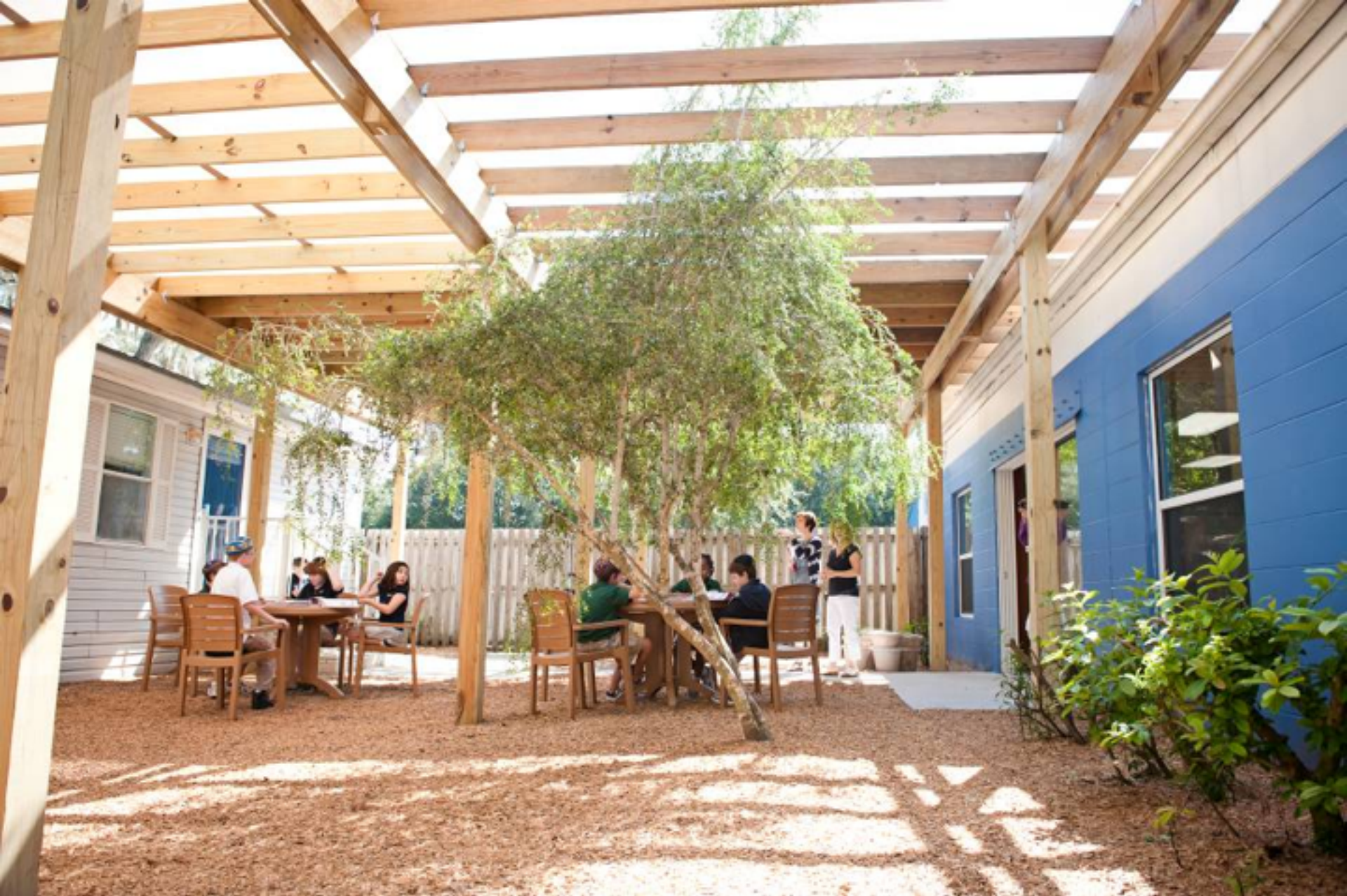
AFTER: This image shows a new trellis that connects the renovated intermediate school (previous photo) with the existing library building. The sheltered area between the two buildings now becomes another great space for outdoor learning. Also note how the entire face of the building has been opened up via glass doors and picture windows
